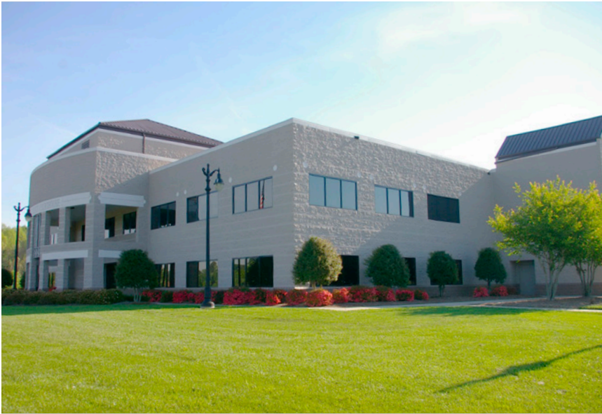
Wilkes County Courthouse worked with Daikin's Service Team to evaluate cost savings and efficiency of a 20-year old chiller versus new air-cooled chiller.
