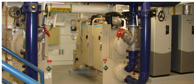
The Daikin WMC Chiller is the quietest chiller in its size range with sound pressure levels as low as 76 dBA per AHRI Standard 575.
